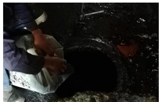
Figure 1: Blending of waste plastic with bituminous binder (upscaling)
