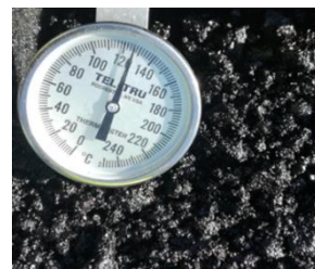
Figure 4: Temperature verification of asphalt mix
