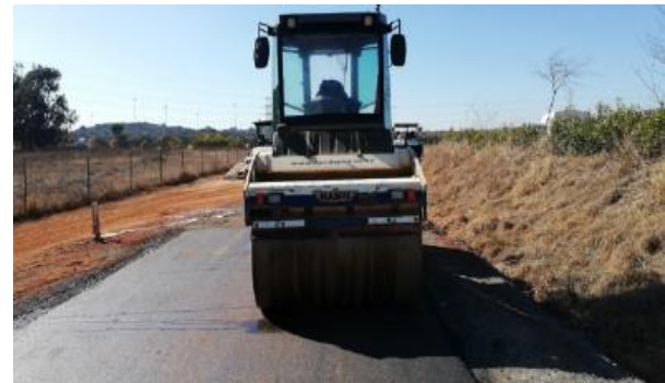
Figure 3: Asphalt compaction and adequate rolling practice
