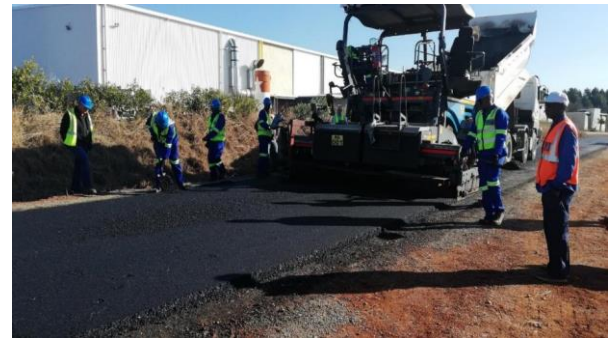
Figure 2: Paving of asphalt test section
