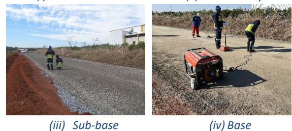
Figure 4: In-situ testing of constructed pavement layers
