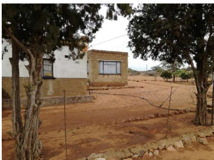
Figure 45: Clean premises around the houses in Matshelapata Source: Researchers
